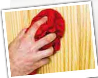
**1.** Make sure all surfaces are clean, dry and free from grease and loose or flaking material.
