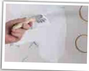
2. Stir well before use and apply Johnstone's Paint to Block Stains by brush or roller. Ensure that an even coat is applied, covering the stain and a surrounding area of 20cm to ensure maximum containment.
