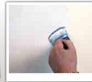
2. Apply an even coat of Johnstone's Paint to Cover Damp. Ensure the affected area is covered completely.
